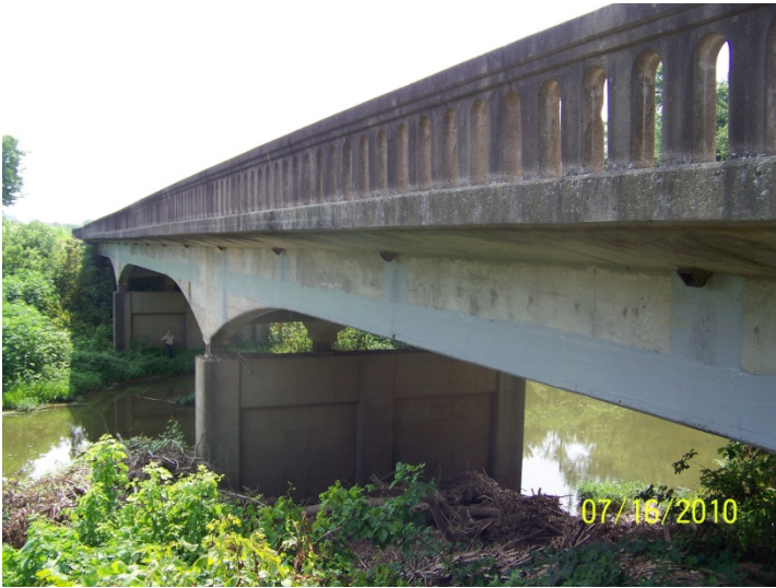
Bridge over Cartwright Creek
