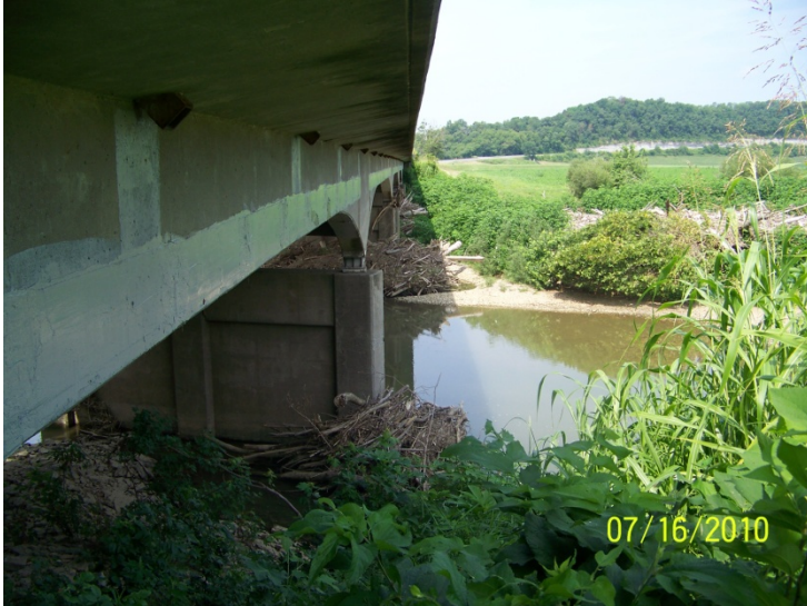
Under Bridge over Beech Fork
