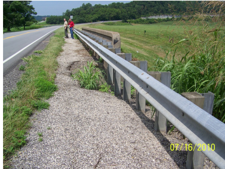
Headwall at Culvert (Roadway Drainage Problems)
