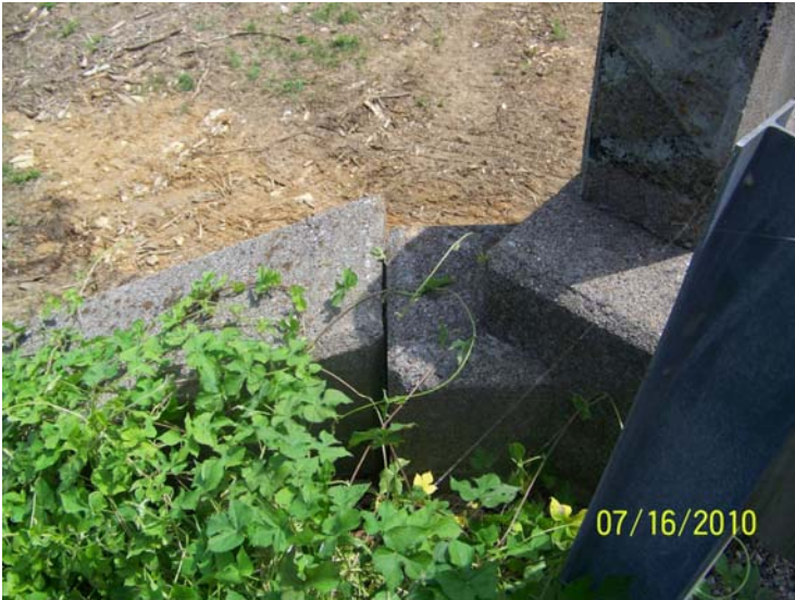
Headwall Separation at Culvert
