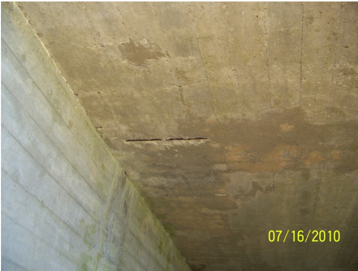
Top of Culvert
