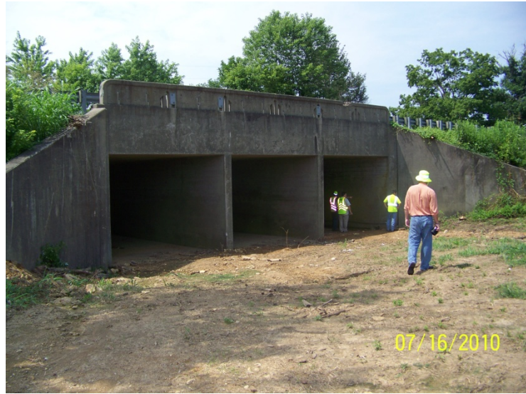
Three Span Culvert (Beech Fork Overflow)
