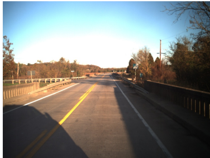
Bridge Over Beech Fork East Approach
