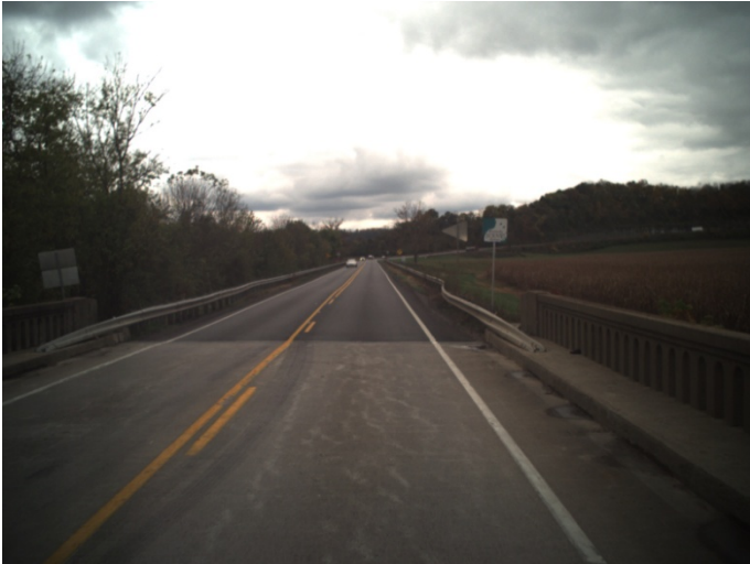
Bridge Over Beech Fork West Approach
