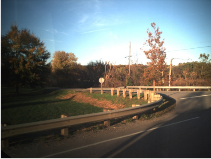
Croakes Station Road
